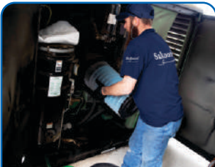
Equipment Installation & Service
